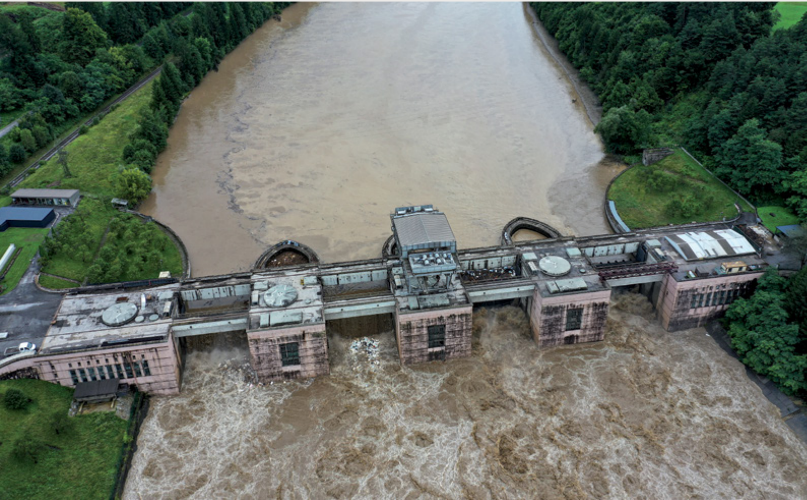
Hydroelectric power plant hit by flood, suffering direct damage.
